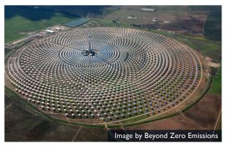
Spain's Gemasolar solar thermal plant uses molten salt storage to run 24 hours per day
