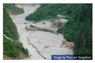
Boulders brought down by the collapse of a mudslide dam created a flash flood in the Bhagirathi River destroying the Vishnuprayag power station in Uttarakhand, India. June, 2013
